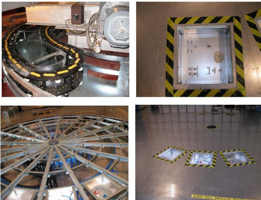
Figure: Principle of energy chain
